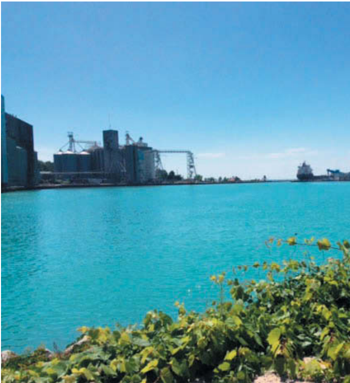
This is the Port of Goderich Ontario on the eastern side of Lake Huron and the buildings and apparatus around the port serve the salt industry.
